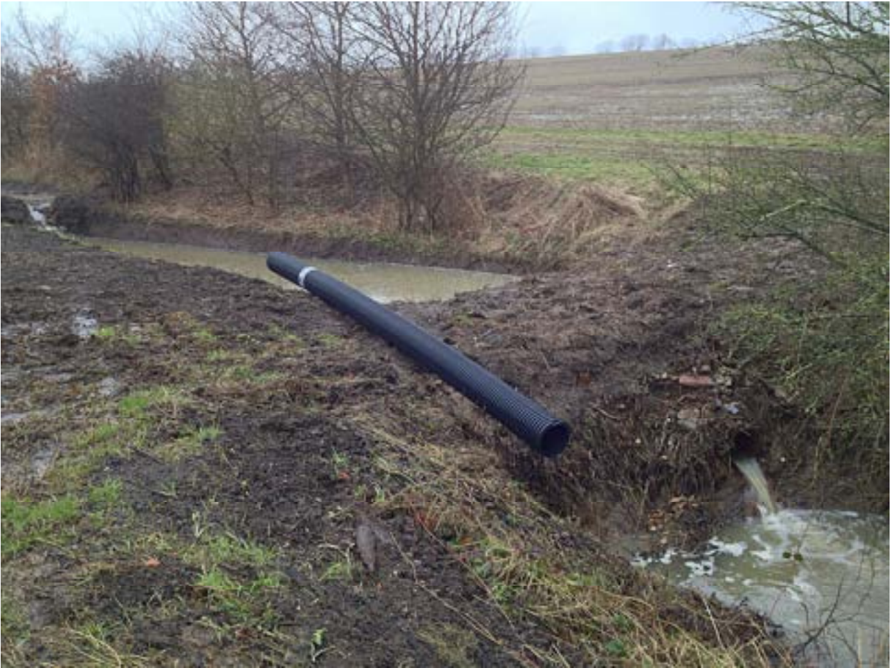
Figure 56. Large earth banded ditch interceptor under construction.
