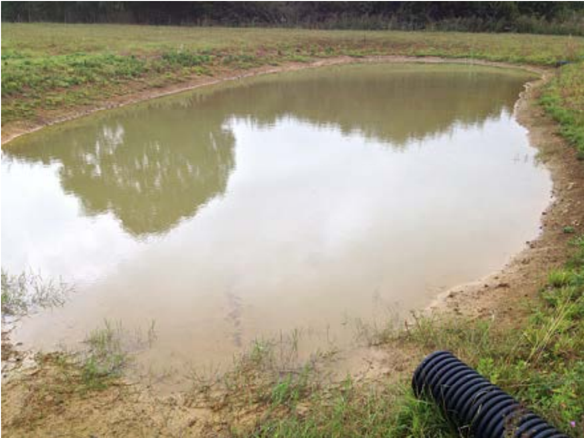
Figure 55. Detail of inlet pipe in a flood detention pond on the Eye Brook (downstream of detention pond in Figure 4). The outlet pipe is visible at the top right of the photograph.
