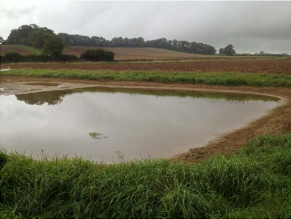
Figure 54. Flood storage basins. This flood storage basin detains water temporarily from the ditch draining the arable area behind the site, including the land upslope to the woodland.
